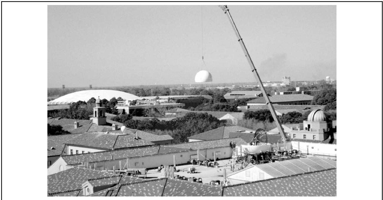
Figure 11. Mounting the RADARSAT SAR antenna on top of the Howe-Russell Geoscience Building for CSI's Earth Scan Laboratory.
