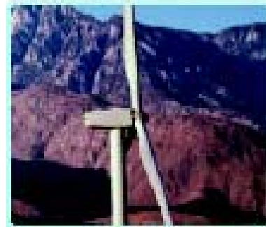
Whitewater Hill California 60 MW
