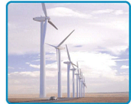
Rock River Wyoming 50MW
